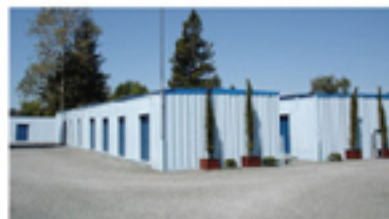
Full access for large trucks
